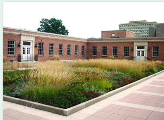
Intensive GreenGrid with concrete curb and concrete pavers on pedestals
