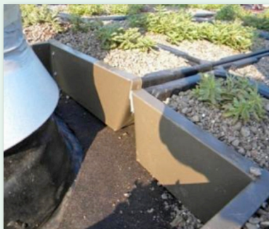
Modules cut and flashed to fit
