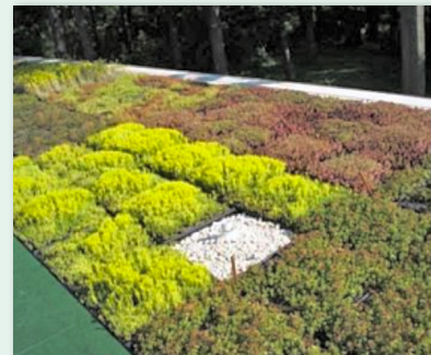
Full module-sized void space left around penetration and filled
