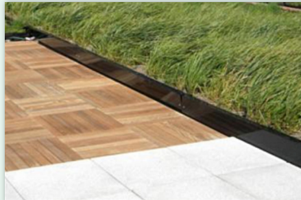
Painted steel trim with Ipe and concrete pavers on pedestals
