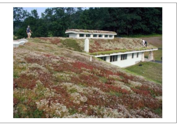
Fig. 6. Extensive green roof Life Expression Wellness Center, Sugar Load, Pennsylvania, USA (C 2005, Roofscapes, Inc., used by permission; all rights reserved)
