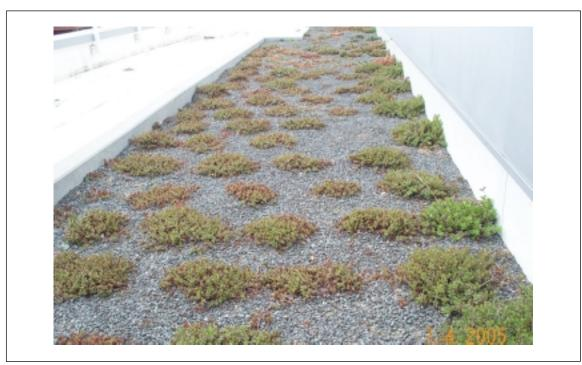
Fig. 5. Extensive green roof with sedums (courtesy of Genzyme Corp.)
