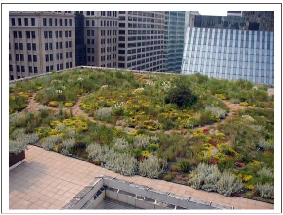
Fig. 4. Extensive green roof, Chicago City Hall, Chicago, Illinois, USA (C 2005, Roofscapes, Inc., used by permission; all rights reserved)
