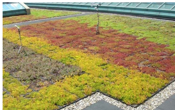
Figure 1: Photograph of the green roof modular system after one year showing above-grade monitoring stands
