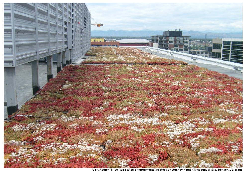
A 19,200 square foot accessible, extensive green roof installed on the new EPA headquarters (2006). Tests have shown an approximate 40% decrease in heat transmitted through the roof compared to the control roof (next door) and an approximate 85% stormwater retention rate for all ½-inch or less storm events.
