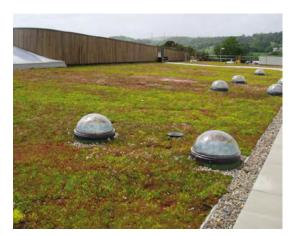
Figure 7: Extensive green roof
