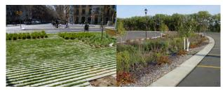
Permeable pavements (left) and biofiltration (right)
