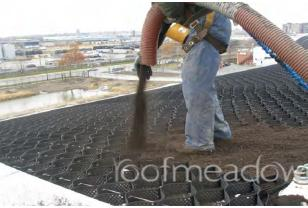
Green roof contractors using a pneumatic blower to install the growing medium
