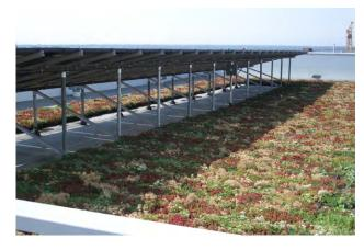
Photovoltaics installed on the United States Environmental Protection Agency Region 8 Headquarters, Denver. Colorado
