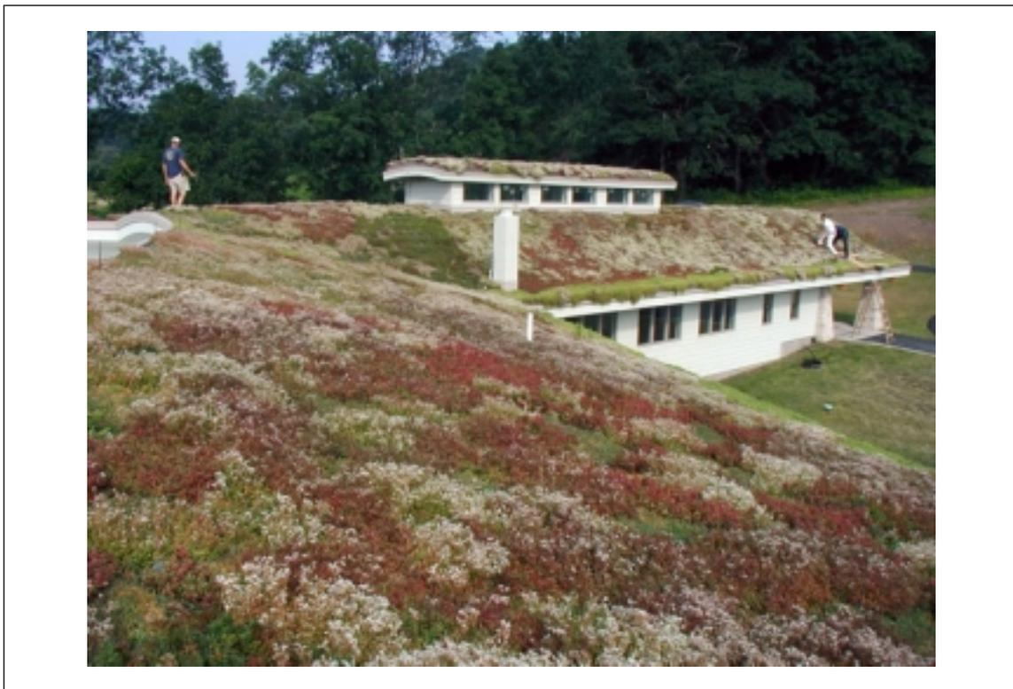
Fig. 6. Extensive green roof Life Expression Wellness Center, Sugar Load, Pennsylvania, USA
