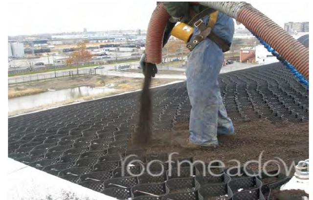
Green roof contractors using a pneumatic blower to install the growing medium
