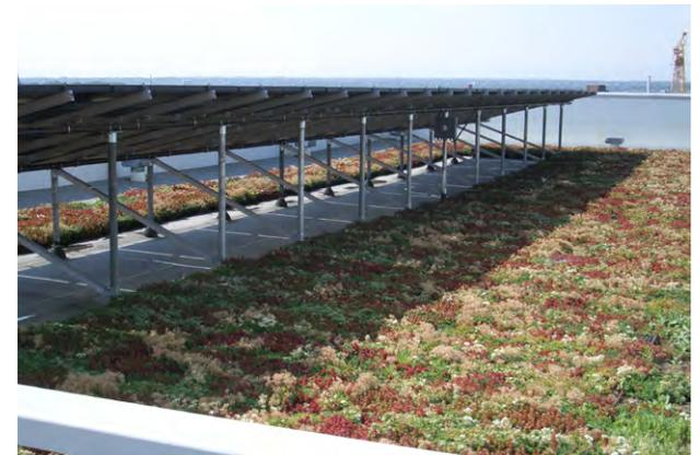
*Photovoltaics installed on the United States Environmental Protection Agency Region 8 Headquarters, Denver, Colorado*
