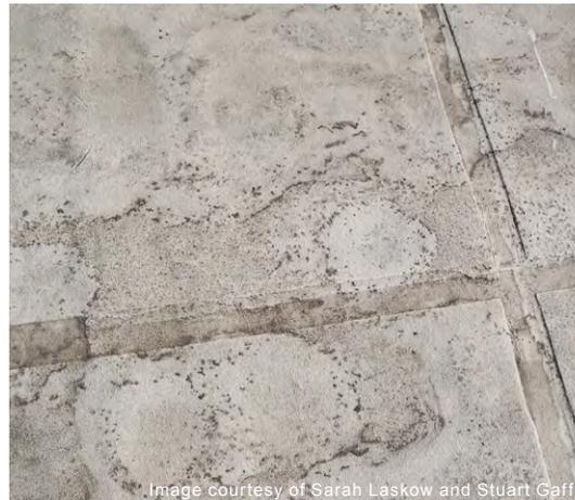
Figure 9: A clean white roof (top) and debris and particulates deposited on a white roof in New York City (bottom)
