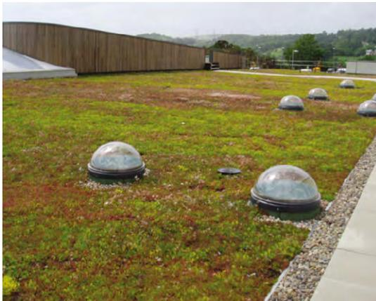
Figure 7: Extensive green roof
