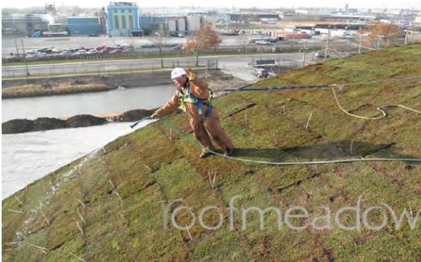
*Irrigating a sloped green roof during the establishment period*
