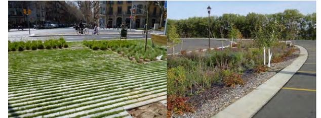
Permeable pavements (left) and biofiltration (right)
