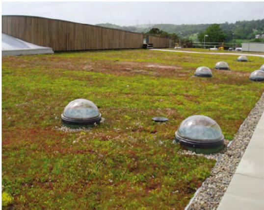
Figure 7: Extensive green roof
